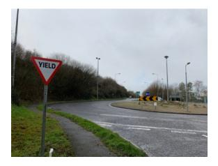
Location 3 - N28/Unclassified Road Roundabout Direction Take 1st Exit At The Roundabout Visual inspection indicates that road widening on central island is required.
